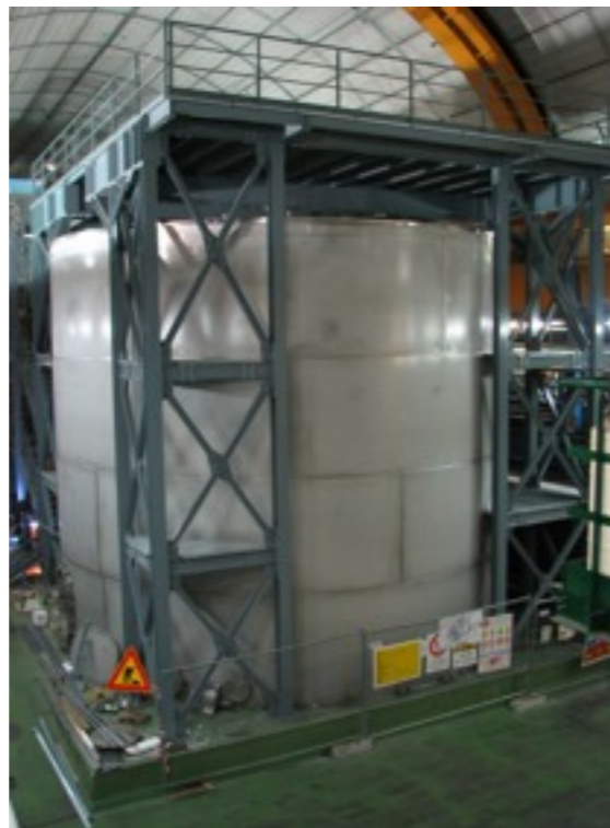
Water tank (July 2008)
